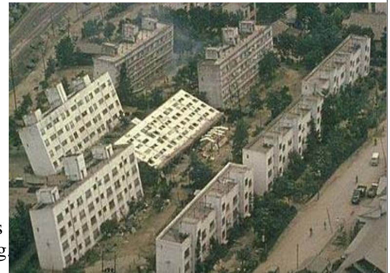
Liquefaction after the 1964 Niigata earthquake, Japan
