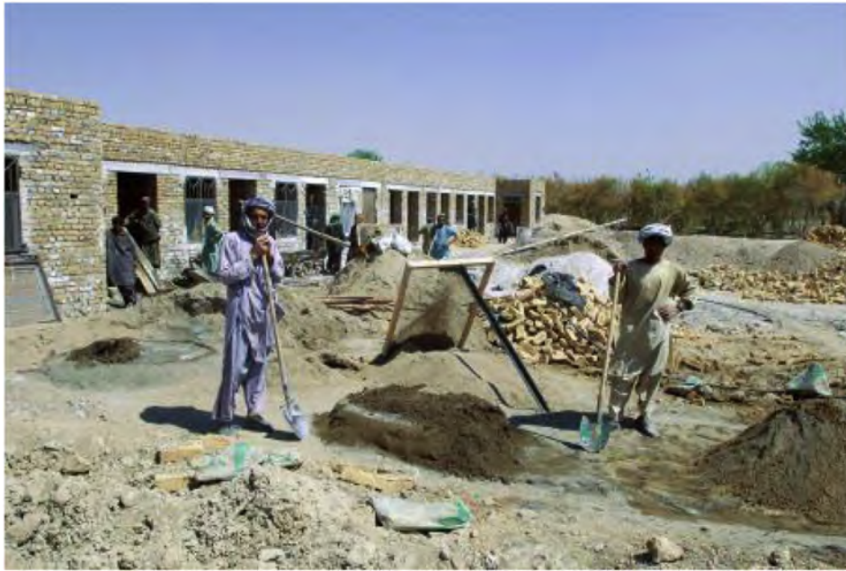
Fig. 2. CERP “cash-for-work” scheme to rebuild houses in Taroke Kalacha. Source: U.S. Defense Video & Imagery Distribution System.
